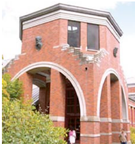
LORRY I. LOKEY SCIENCE COMPLEX, WILLAMETTE HALL
